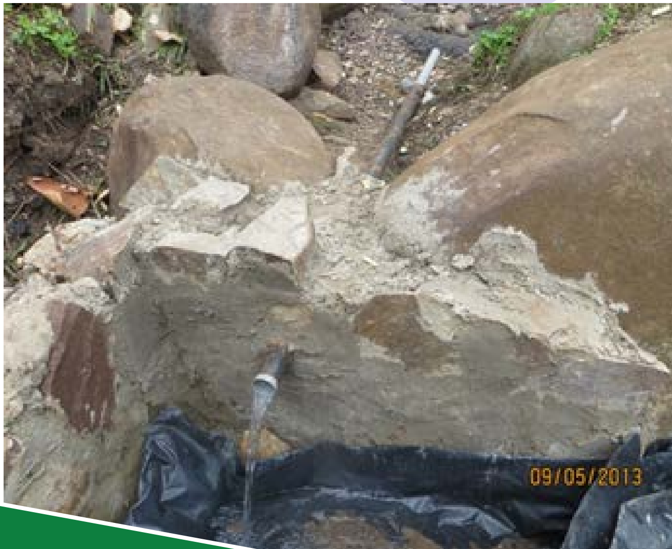
The protected water source after rehabilitation
